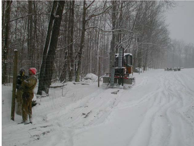
Kilgore 11-Acre Deer Exclosure Under Construction
